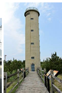
World War II Lookout Tower (Fire Control Tower No. 23)
